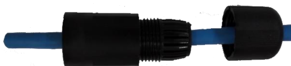
Figure 2-27 Cabling and Ethernet plug making
